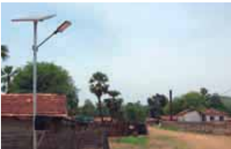
Solar photovoltaic street lighting
