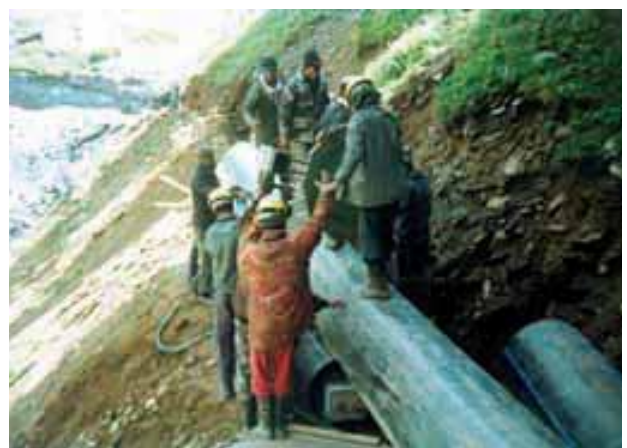
Installation of PE pipe along the Himalayan slopes in HP
