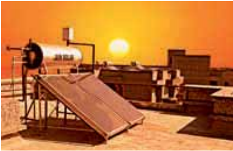
Solar water heating system
