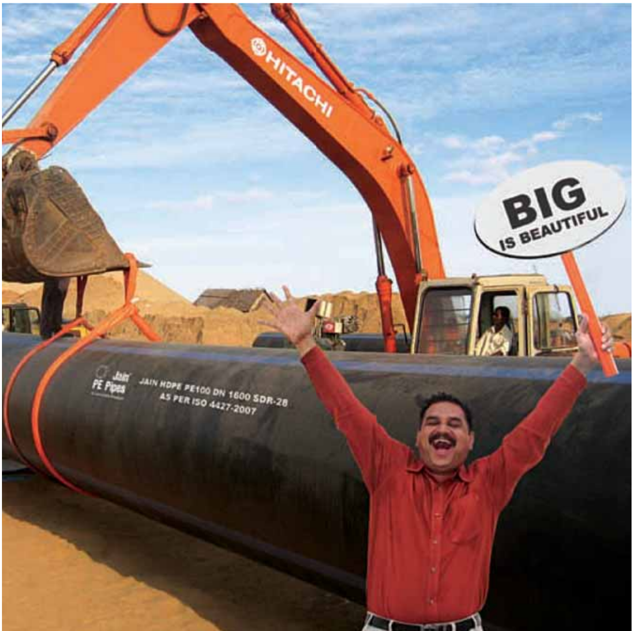
1600 mm PE Pipe under installation off the Chennai coast
