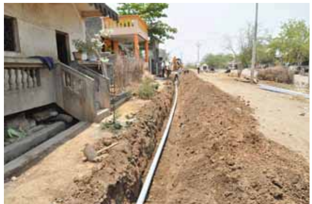
Conveying water; laying a pipeline in the Shirsoli Panchayat for drinking water
